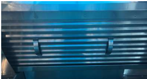
Illegally modified filter
