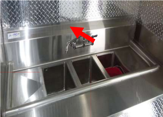
Caulking smooth and easily cleanable
