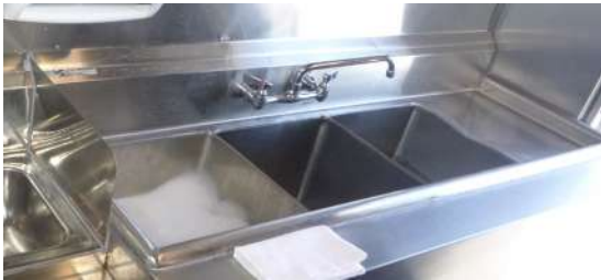
Only one drain board
