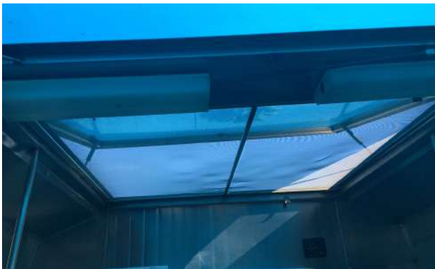
Properly screened overhead opening
