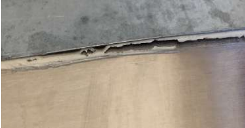
Cracked caulking
