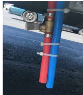
Drain valve must be rigid.
