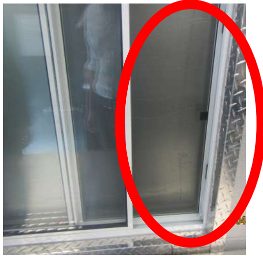
Service window larger than 18x18 inches
