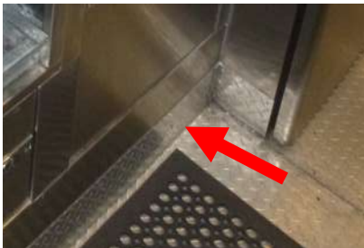
Equipment properly sealed to the floor
