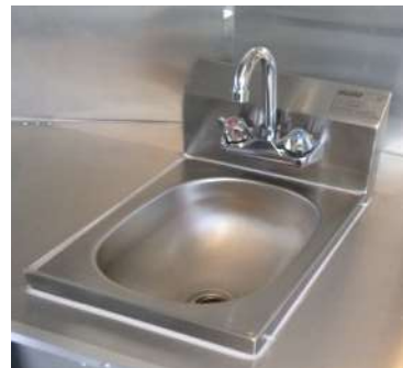
Hand sink does not meet the minimum size requirement and needs splash guard
