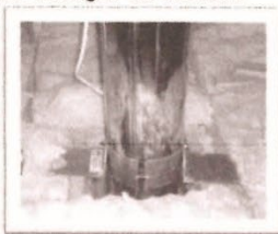
PICTURE 3-4. INSTALL ROOF SUPPORT
