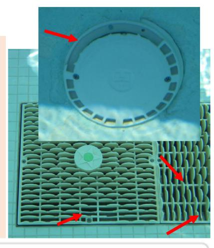
WARNING! - Failure to remove pressure test plugs and/or plugs used in winterization of the pool/spa from the suction outlets can result in an increased potential for suction entrapment as described above.
