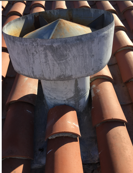
View of Roof Flashing (HA#04)
