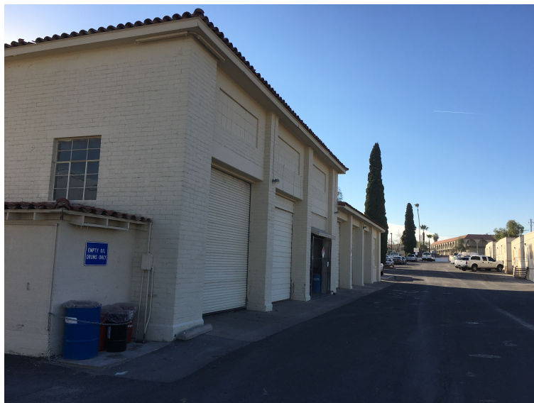
View of Building F Facing Southwest
