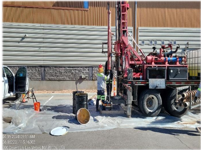
Figure 2.6-2 Geotechnical Drilling
